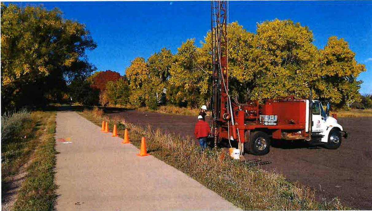
Photo 1. View looking at drilling Boring B-1.
